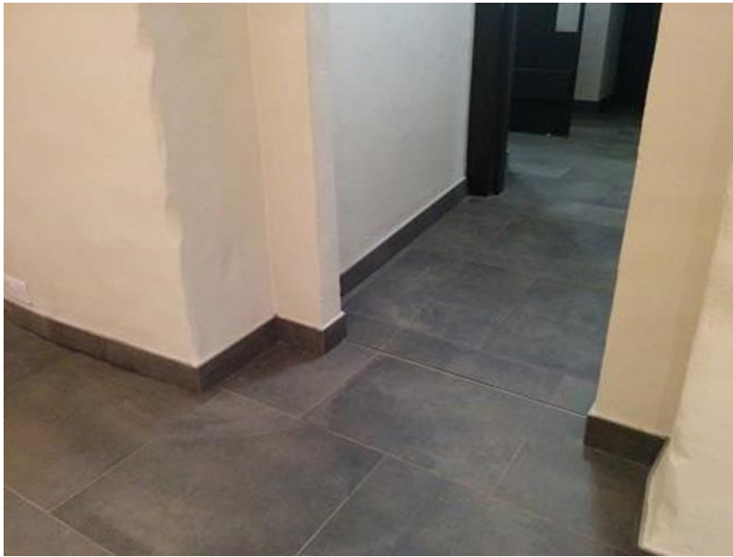
Image 15: Upwards slope to toilets
