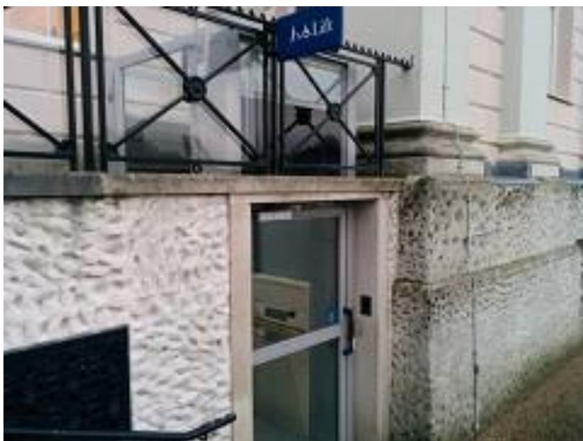
External Platform Lift on east side of museum
