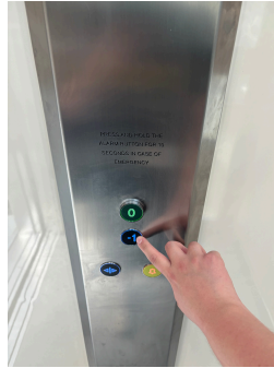
You have to keep holding the button for the lift to move up or down.
