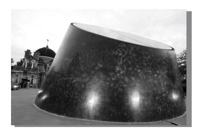
The centrepiece here is the large metal structure below which is the planetarium. One wall points directly overhead. One wall is slanted at an angle equal to our latitude (51.5°) and points to the North Star (Polaris). The cone is sliced at an angle equal to 90° - 51.5° and represents the celestial equator (the extension of the Earth's equator out into space). It is aligned north-south so it acts as a giant sundial.
